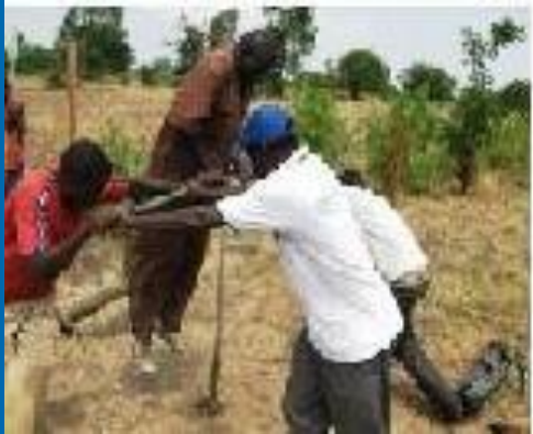
Construction of piezometers
